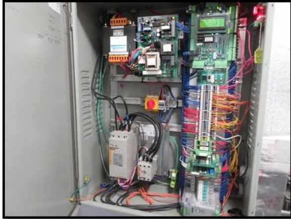
Figure 5 – Elevator Controls
