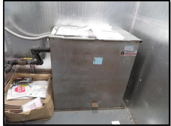
Figure 6 - Elevator Pump
