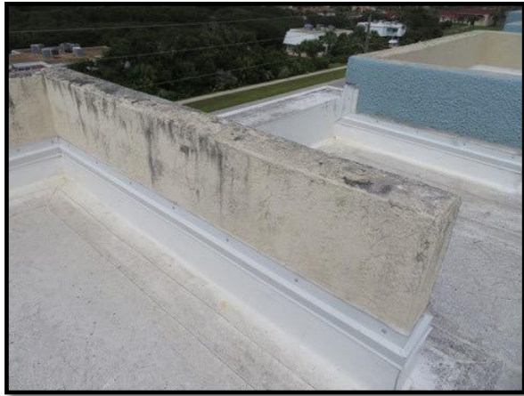
Figure 1 – Rooftop Parapet Wall
