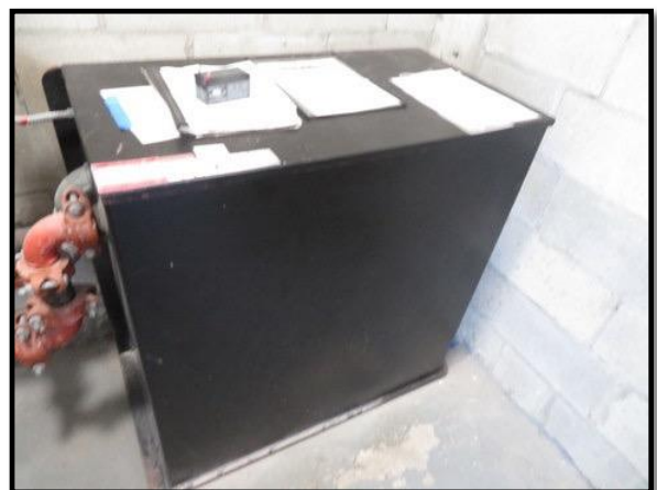
Figure 4 – Elevator Pump
