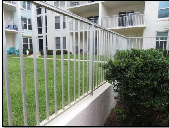
Figure 1 – Pool Area Railing
