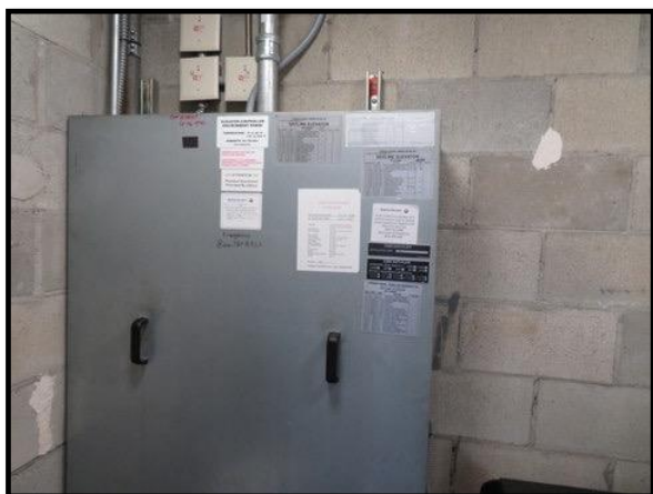
Figure 3 – Elevator Controls
