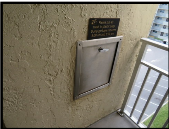
Figure 21 Trash Chute Door
