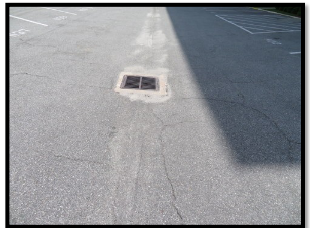
Figure 42 Storm Water Catch Basin
