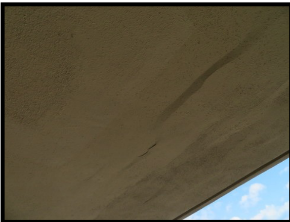
Figure 15 Top Breezeway Ceiling Bubbling
