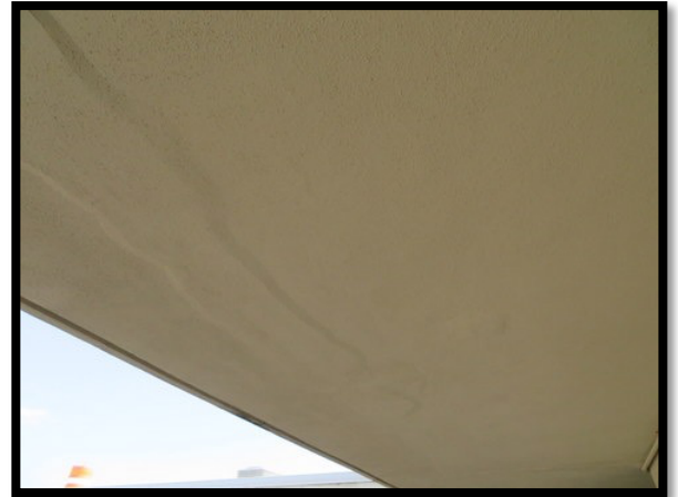
Figure 17 Window Sill Crack
