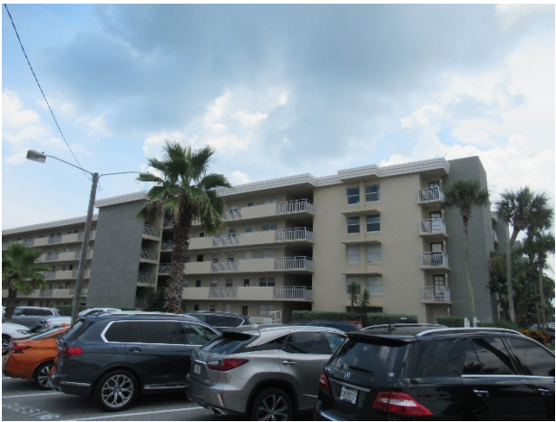
Building north side
