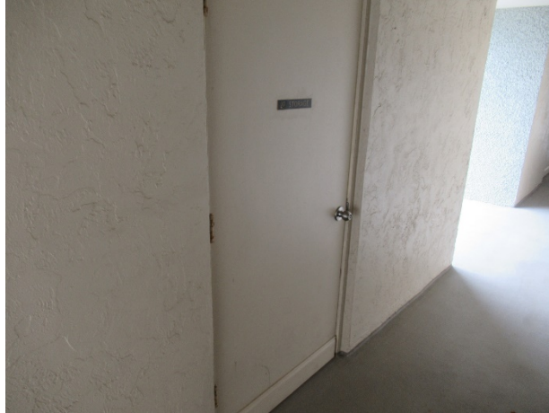
Typical storage room door
