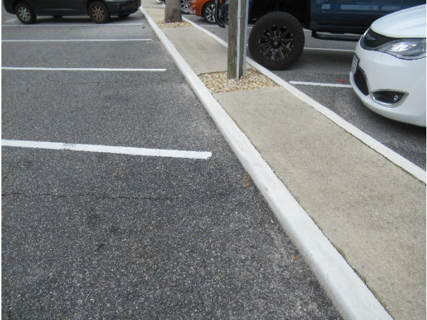
Typical concrete curbs
