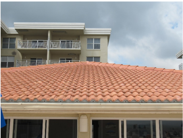
Typical concrete tile roof
