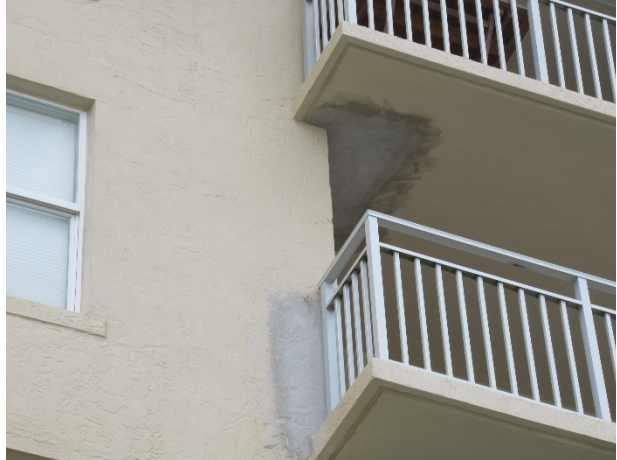
Balcony with recently repaired concrete
