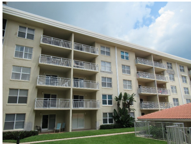
Building south side
