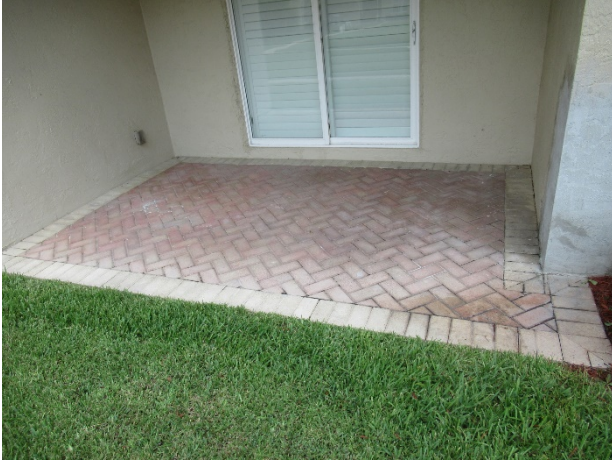
Typical paver patio
