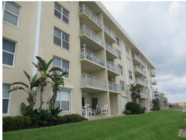
Building east side
