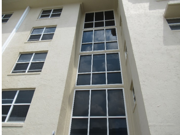
Windows at the breezeways and the laundry rooms
