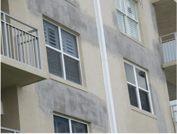
Recent stucco repairs
