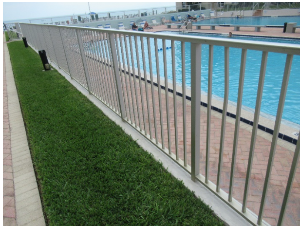
Pool fence overview
