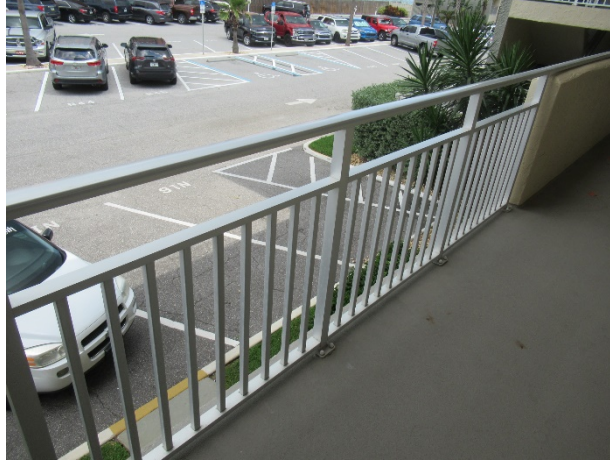
Typical railings at the breezeways and balconies
