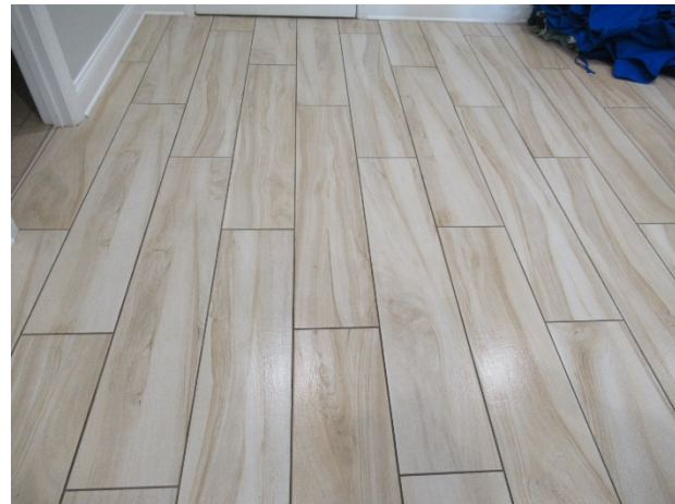
Tile Flooring replaced in 2019
