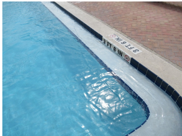
Plaster and tile finishes
