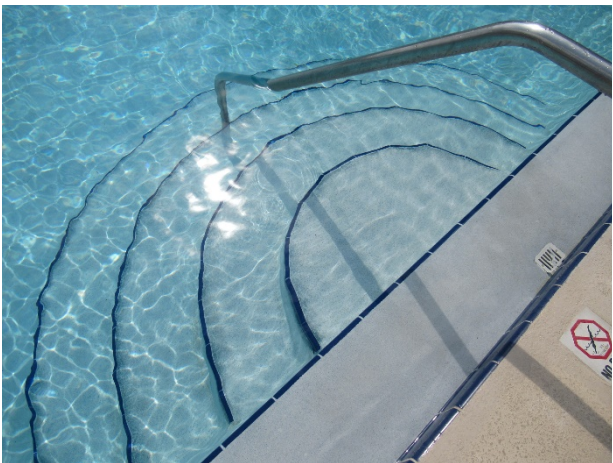
Plaster and tile finishes
