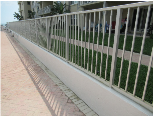
Pool fence overview
