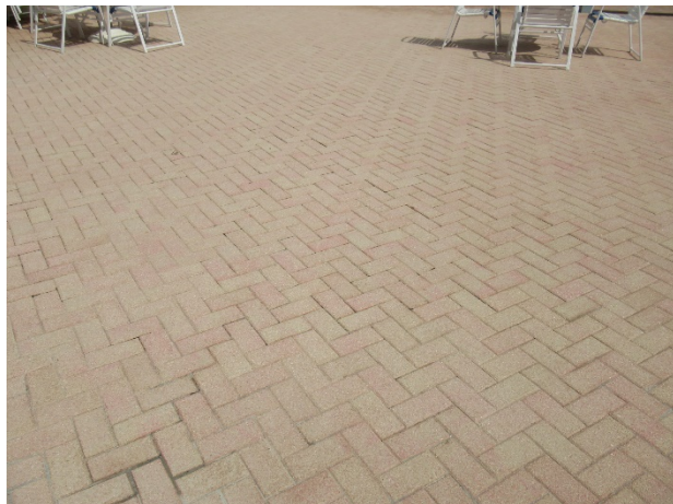
Pool deck pavers
