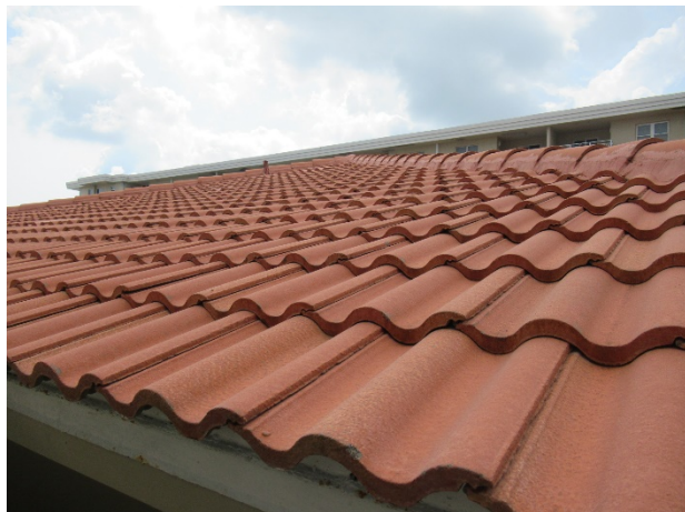
Typical concrete tile roof
