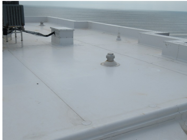
Thermoplastic roof overview
