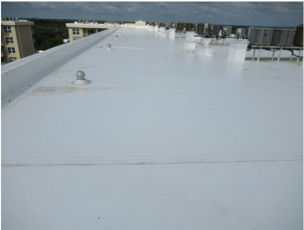
Thermoplastic roof overview
