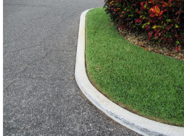
Typical concrete curbs
