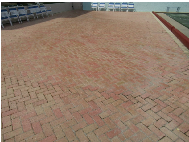
Pool deck pavers
