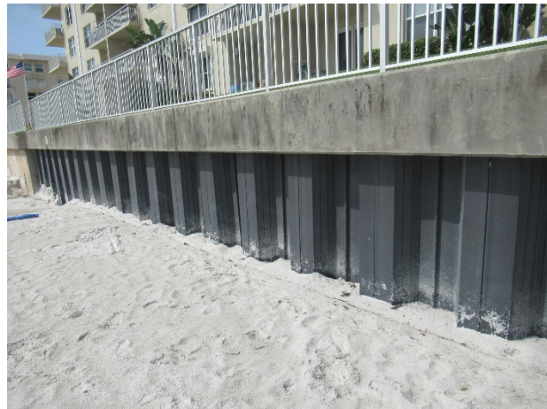
Vinyl section of bulkhead
