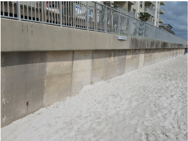
Original concrete bulkhead
