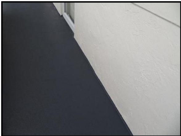
Figure 3 – Typical Breezeway Floor
