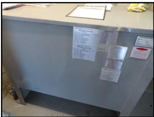
Figure 1 – Elevator Pump
