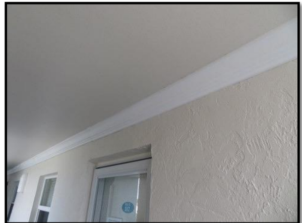
Figure 4 – Covered Wall to Ceiling Joint
