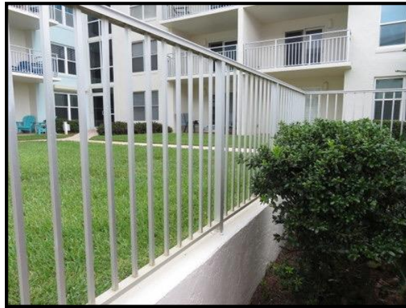
Figure 1 – Pool Area Railing
