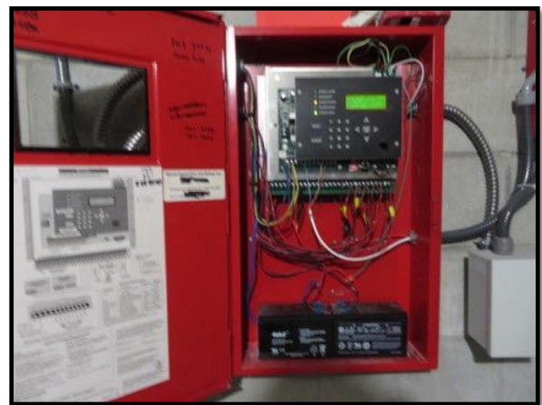
Figure 2 - Control Panel
